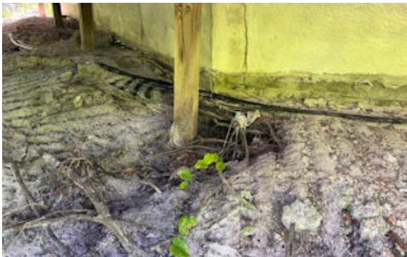
Soil stabilized under wall and crack sealed
