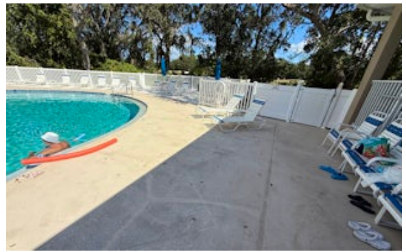
Stabilization of pool deck
