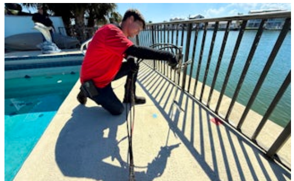
Pool Deck Stabilization
