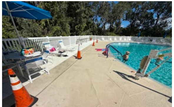
Stabilization of pool deck
