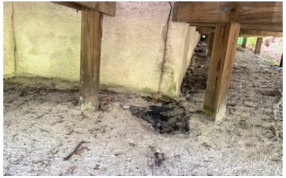
Soil Stabilized under wall and crack sealed
