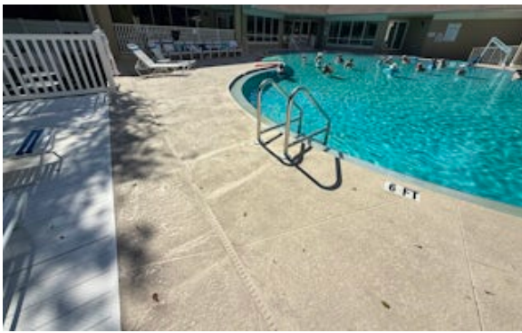
Stabilization of pool deck
