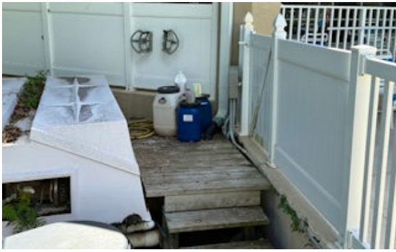
New PVC drain line from gutter under equipment out to swamp area
