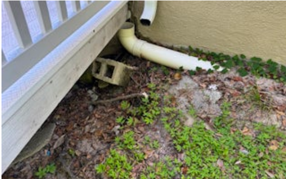
Bring in soil and mount catch basin underneath gutter and ran out to lower elevation
